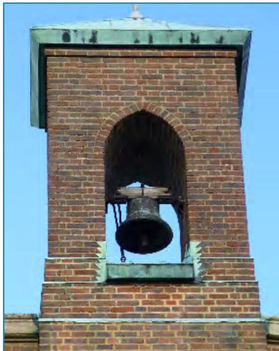
After many years of constant use and exposure to the elements, it has now become impossible to ring the bell. An inspection by Whites of Appleton in August (delayed due to the exigencies of COVID restrictions) revealed that the wooden headstock is badly decayed, the chiming lever broken and much of the metalwork corroded.
