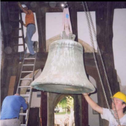
The old tenor bell being lowered from the tower
